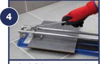
Apply light pressure, push down the handle and score the full length of the tile.
