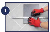
Measure & mark a visible line along the length of the tile
